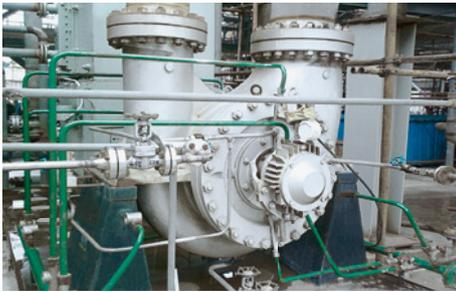
Fujian Refining & Petrochemical Co., Ltd. in China applies a BB2 pump for propane de-asphalting. The shaft seal is an EagleBurgmann **SHV1/102-PTA1/2**. Configuration 2CW-CW, piping plans 21+52. Operating conditions:  $p = 73 \text{ barg (1,059 PSIG)}$ ;  $t = 165 \text{ }^\circ\text{C (329 }^\circ\text{F)}$ ;  $n = 2,970 \text{ min}^{-1}$ .
