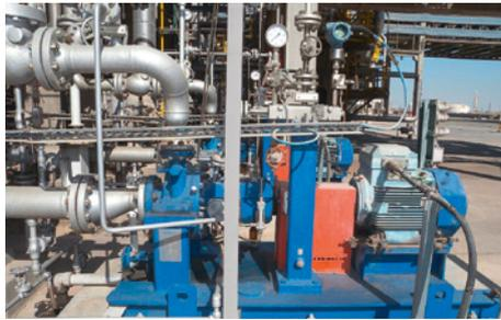
De-ethanizer pump in a LPG fractionation unit of the ENOC refinery, U.A.E., equipped with an unpressurized dual EagleBurgmann **sealing system to API 682**. Configuration: 2CW-CS, piping plans 14 and 76. Operating conditions: p = 36 ... 39 bar (522 ... 566 PSI); t = 1 °C ... 43 °C (34 °F ... 109 °F); n = 2,933 min<sup>-1</sup>. Medium: LPG. The MTBF has improved drastically since installation.
