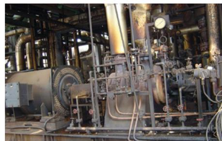
Kochi Refineries Ltd., India applying in their visbreaker unit EagleBurgmann metal bellows seals **Y14D52C** with a supply system to API 682 Plan 32 + 62 in an Ebara centrifugal pump. Operating conditions:  $p = \dots 8.9 \text{ bar (129 PSI)}$ ;  $t = 247 \text{ }^\circ\text{C (477 }^\circ\text{F)}$ ;  $n = 1,780 \text{ min}^{-1}$ ;  $p_1 = 75 \text{ mm (2.95")}$ . Medium: vacuum residue.
