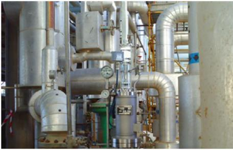
EagleBurgmann mechanical seals are installed in demethaniser reboiler pumps from Thompson Byron Jackson at the Santos-owned Moomba gas plant in South Australia. EagleBurgmann solved the challenges with its seal type **H75KF-D** and a supply system to API 682 Plan 53C. Operating conditions:  $p = 36 \text{ bar}$  (522 PSI);  $t = -20 \text{ }^\circ\text{C} \dots +38 \text{ }^\circ\text{C}$  (-4 °F ... +100 °F);  $n = 1,480 \text{ min}^{-1}$ . Media: light hydrocarbons.
