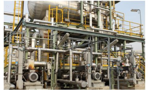
The ENI refinery in Sannazzaro De' Burgondi, Italy, operates a Finder centrifugal pump in its gasification unit. The pump is sealed by EagleBurgmann **HRKS4-DF/58** mechanical seals. Operating conditions: p = 16.08 ... 19.93 bar (233 ... 289 PSI); t = 238 °C ... 263 °C (460 °F ... 505 °F); n = 2,955 min<sup>-1</sup>; d1 = 80 mm (3.15"). Medium: carbon slurry.
