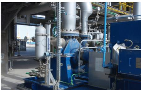
Stripper reflux pumps within the naphtha hydro treater unit of the ENOC refinery in Dubai are fitted with EagleBurgmann **H75VKS20/105** mechanical seals and supplied to API 682 Plan 11. Operating conditions:  $p = 11.77 \text{ bar}$  (25 PSI);  $t = 43 \text{ }^\circ\text{C}$  (109 °F);  $n = 1,485 \text{ min}^{-1}$ ;  $d1 = 80 \text{ mm}$  (3.15"). Media: hydrocarbons.
