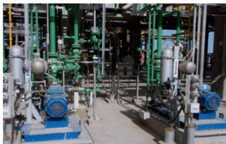
In the ENOC refinery in Dubai, U.A.E., LPG pumps are sealed by EagleBurgmann **H75VKS20/85** dual tandem face-to-face mechanical seals. Applied API piping plans: 11 + 53B. Operating conditions:  $p = 17.75 \text{ bar}$  (257 PSI);  $t = 43 \text{ }^\circ\text{C}$  (109 °F);  $n = 2,950 \text{ min}^{-1}$ ;  $d1 = 60 \text{ mm}$  (2.36"). Media: hydrocarbons.
