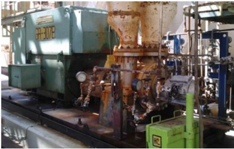
In the alkylation plant of the refinery of Salina Cruz, Oaxaca, Mexico, our **H74-D/85** functions as a dual seal for between bearings pumps from Byron Jackson. Operating conditions:  $p = 9.61 \text{ bar}$  (139 PSI);  $t = 42.3 \text{ }^\circ\text{C}$  (108 °F);  $n = 3,550 \text{ min}^{-1}$ ;  $d1 = 79.38 \text{ mm}$  (3.12"). Media: hydrocarbons + hydrogen fluoride.
