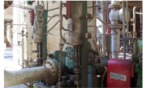
Since 2001, PDVSA (Petroleos de Venezuela) has been using EagleBurgmann seals type **H75K/110** with supply system **TS6050** to API 682 Plan 52 in a Sulzer between bearings pump. Operating conditions:  $p = \dots 4 \text{ bar (58 PSI)}$ ;  $t = 52 \text{ }^\circ\text{C (126 }^\circ\text{F)}$ ;  $n = 3,560 \text{ min}^{-1}$ ;  $d_1 = 80 \text{ mm (3.15")}$ . Media: aromatic hydrocarbons.
