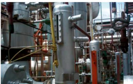
Since 2002, a refinery in Minatitlan, Veracruz, Mexico, has been using the EagleBurgmann **H75K/90** together with a **TS6050** seal supply system and **WDK5120** cooler to API 682 Plan 21 + 52 in a Sulzer centrifugal pump for distillation. Operating conditions:  $p = \dots 17.89 \text{ bar (259 PSI)}$ ;  $t = 247 \text{ }^\circ\text{C (477 }^\circ\text{F)}$ ;  $n = 1,780 \text{ min}^{-1}$ ;  $d_1 = 75 \text{ mm (2.95")}$ . Media: hydrocarbons with traces of  $\text{H}_2\text{S}$ .
