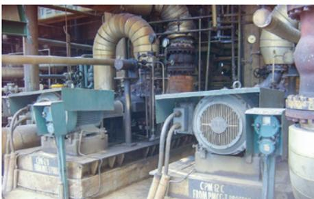
EagleBurgmann seal type **Y14D64TC** with supply system to API 682 Plan 11 and 62 running successfully in a KEPL centrifugal pump in the distillation unit of Kochi Refineries Ltd., India, since 2002. Operating conditions:  $p = \dots 9.6 \text{ bar (139 PSI)}$ ;  $t = 42.3 \text{ }^\circ\text{C (108 }^\circ\text{F)}$ ;  $n = 3,550 \text{ min}^{-1}$ ;  $d_1 = 100 \text{ mm (3.94")}$ . Media: hydrocarbons + hydrogen fluoride
